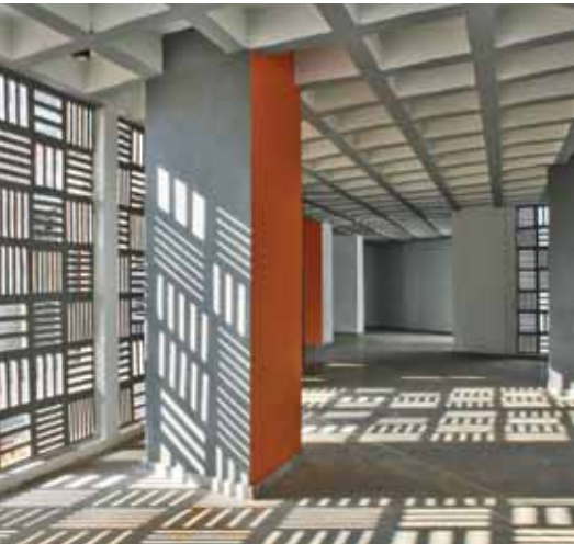
The Science block building is articulated through material modulation as well as the use of elements like slender columns, jaalis and size of openings; the use of the waffle slab not only defines movement within the non-linear spinal corridor but also visually integrates with the flooring and jaali patterns
