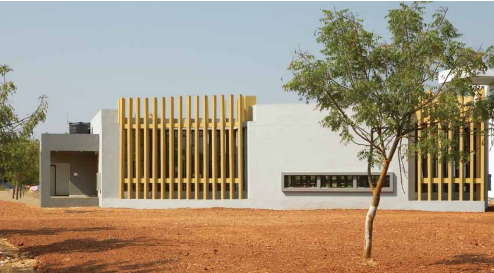
The dining hall is a stark cuboid punctuated by scooping out volumes that design the entry of light into the deep interiors as well as make pockets of landscape possible; these scoops are marked by vertical fins that modulate the entry of harsh light while thin horizontal slits allow for outside views while dining
